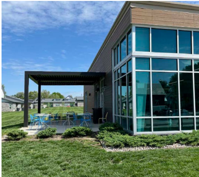
Covered outdoor seating at Public Library.
