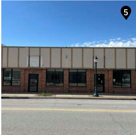
Vacant Office Land Use: Commercial Scale: Small, 1-story
