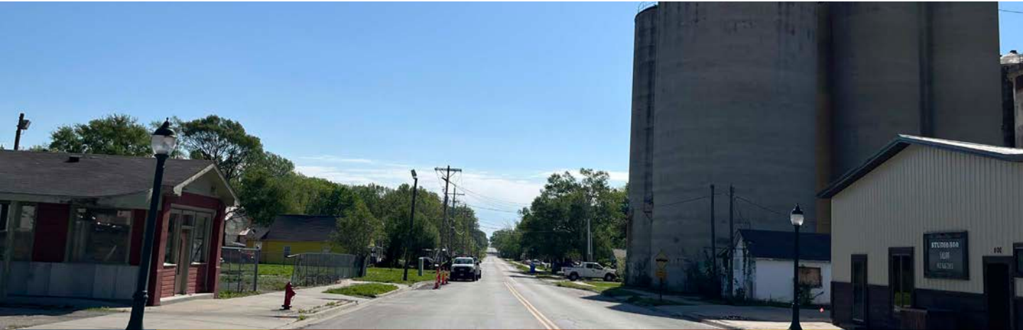
4th Street Existing Conditions (East Transition Zone)
