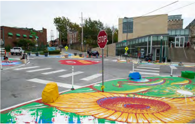
Painted curb extensions slow traffic and reclaim space for pedestrians of all ages, and can be implemented quickly at a low cost.
