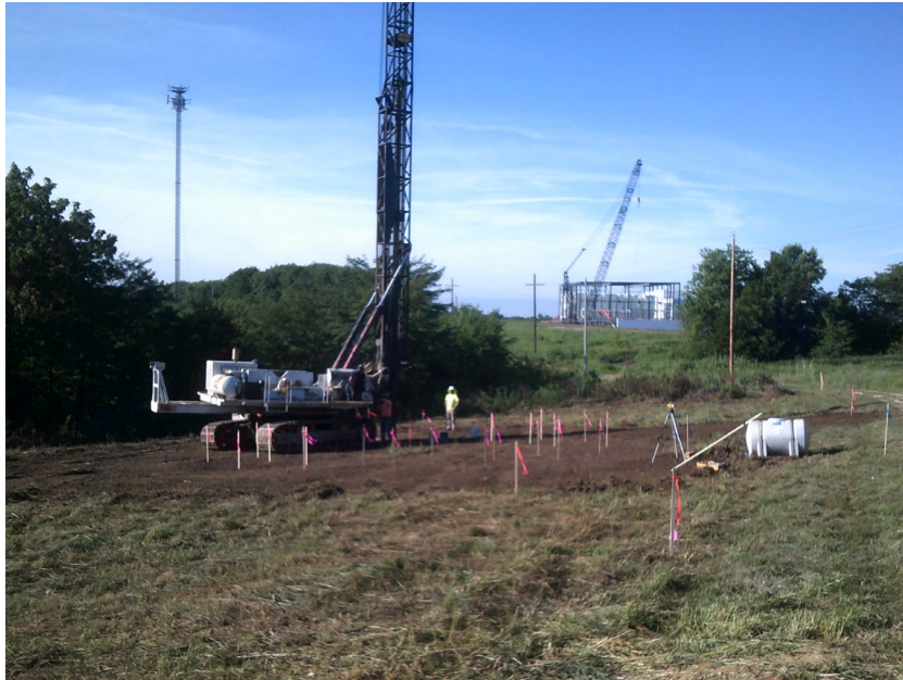
1. Began drilling operations for the drilled shafts.
