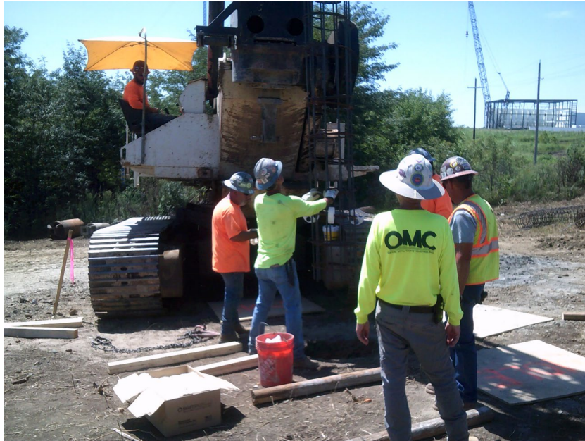
3. Cleaning out hole.
