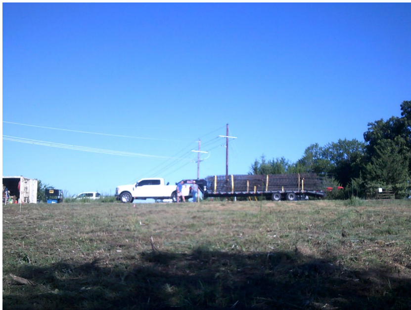
2. Delivered rebar cages already tied.
